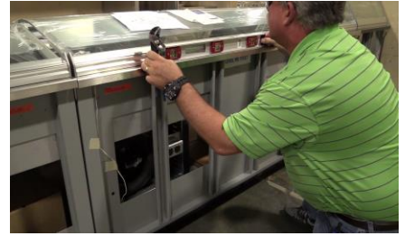
Start leveling with the cold section first. Use level to determine adjustment direction and ensure the top of the unit is parallel to the ground.
