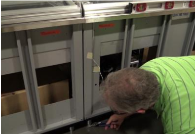
Each unit comes with adjustable feet. Use adjustable pliers to raise or lower the unit as necessary.
