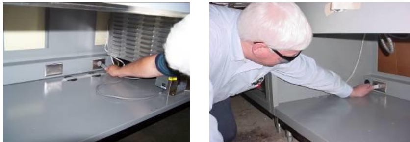
Plugging in the cord for the condenser unit and the hot food unit
