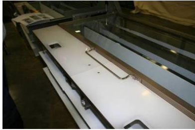
The units are shipped with the day cover in the down position. Raise the day cover and secure with lock before leveling.
