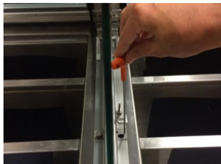
Use end mount adjustment screws and 3/32 Allen Wrench if necessary, to ensure proper vertical position of end glass.
